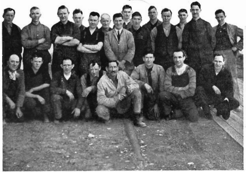
The gang of fitters and fitters' assistants under Mr. Goodyear, who did such excellent work in installing the equipment of the Boiler Shop
