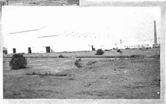
December 23: Exterior of shop complete
