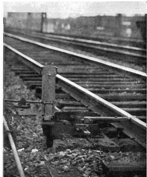
The Arm of a Clayton Fogging Machine Holding a Detonator on the Rail
