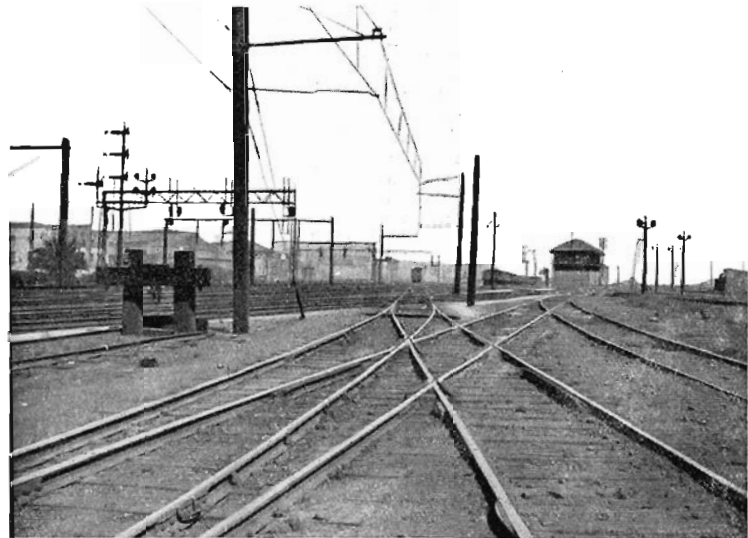
Fig. 3. The diagonal track taken by engines from the Loco. Shed to the Spencer-street platforms. A locomotive is seen in the distance
