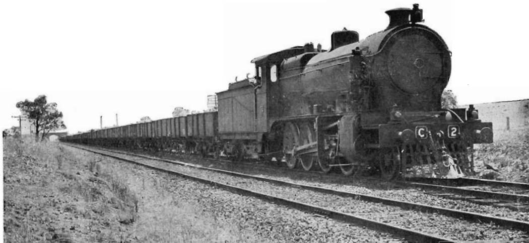
A Modern Wheat Train. The "C" class Engine is hauling 1212 tons of grain
