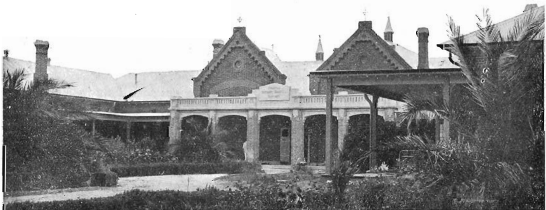
Horsham's New Base Hospital.
