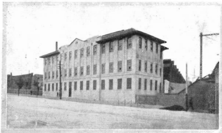
The Melbourne Yard main office. While the city sleeps, a control staff, located here, keeps in close touch with shunter and signalman in the yards below.
