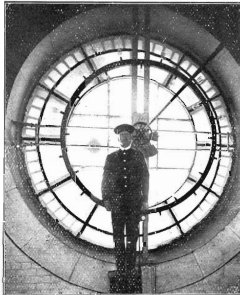
This photograph illustrates the size of Flinders Street Tower Clock Dial
