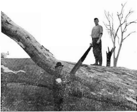
Cutting timber into sleeper lengths
