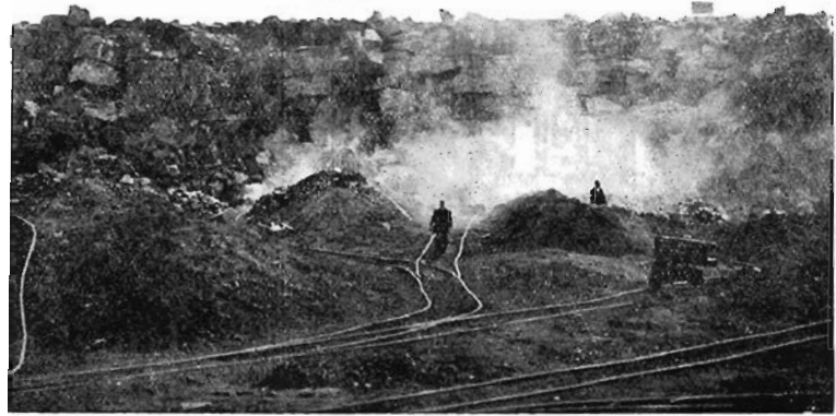
Lighting fuses prior to the mid-day blasting
