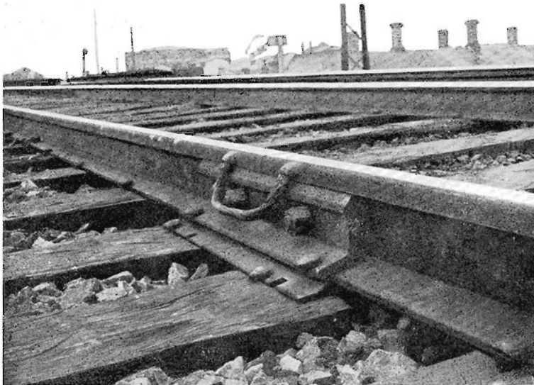
110-lb. rails recently laid on the Clifton Hill Line
