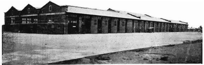
Aviation siding temporary workshop.
