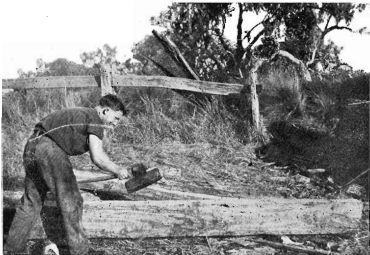
The Finishing Touches
