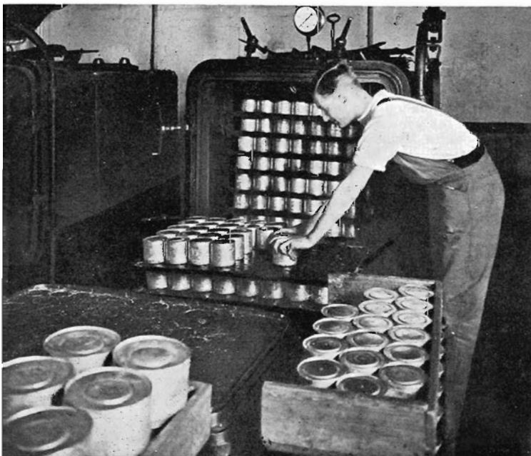
One of the retorts being filled
