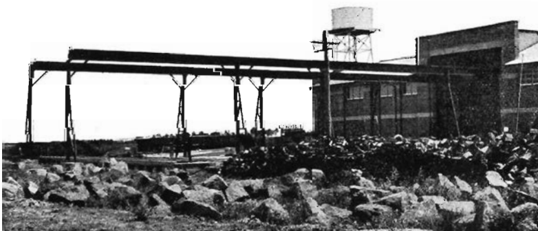
The crane run-way from the aviation store to the siding.
