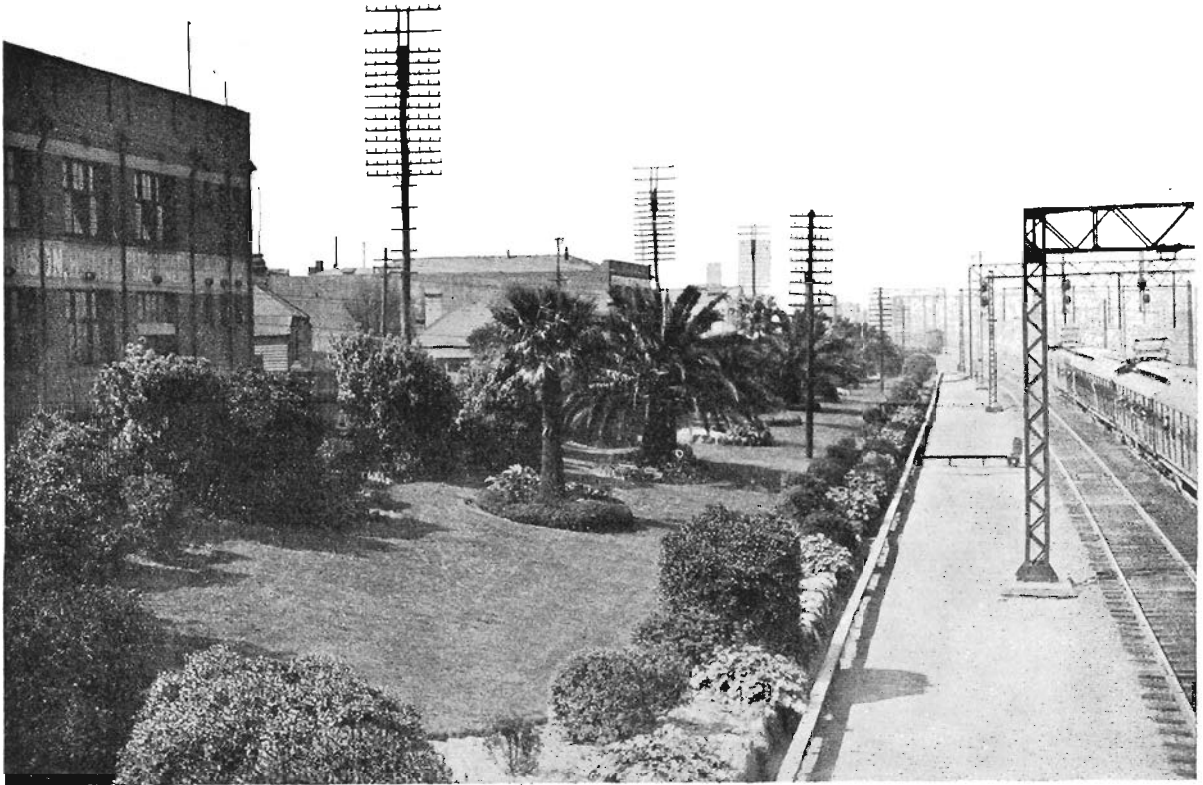
Railway Garden at North Melbourne
