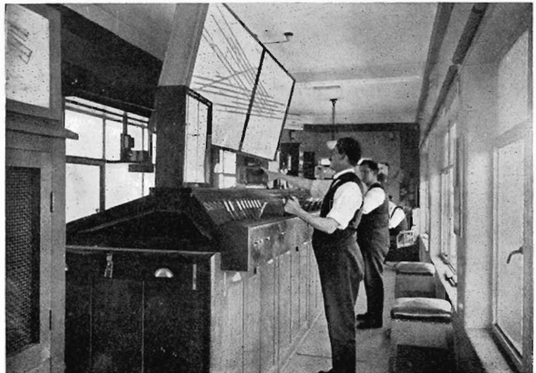
Fig. 1. Interior of Franklin-street Junction Special Signal Cabin
