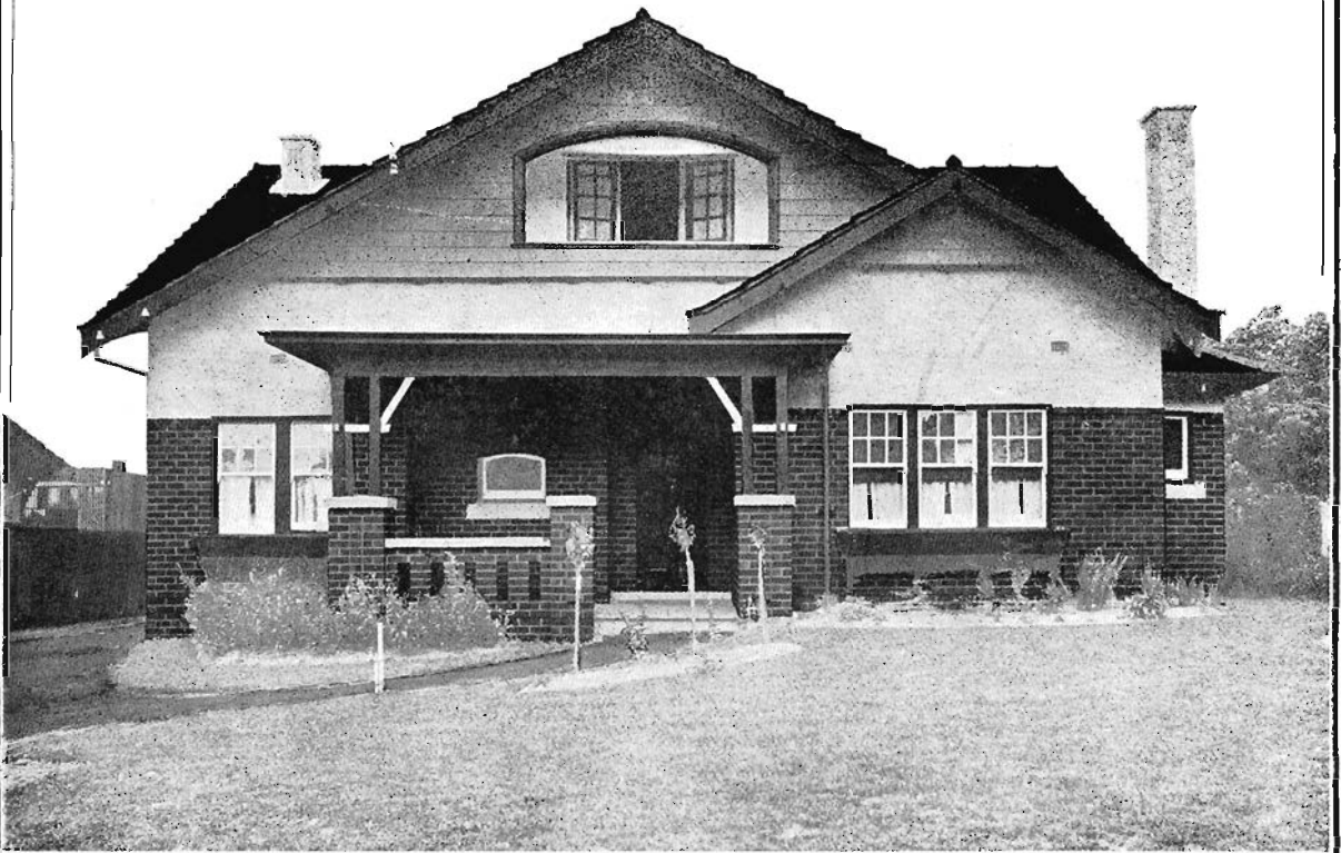
Brick Residence designed and erected for H. Wilson, Esq., Hillcrest Avenue, Kew
